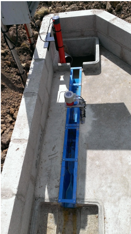
Example: Channel with level/flow-rate and pH monitoring
