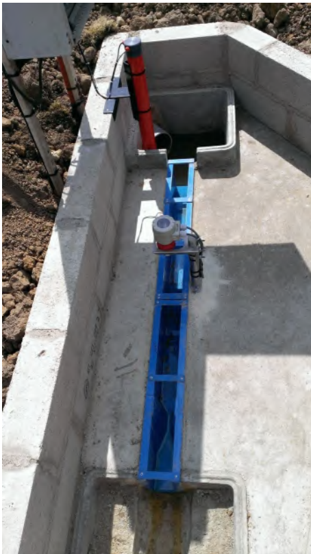
Example: Channel with level/flow-rate and pH monitoring
